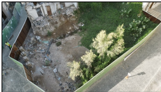
Figure 32. Existing Location of Al-Jilani Zawiya after Demolition. (Source: Author, 2024)
