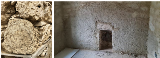
Figure 7. Manqabi stone and Nora as basic material for buildings in Historical Jeddah District (Source: Author, 2024)
