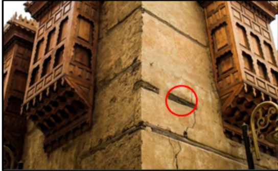
Figure 15. Wood Beams of Historical Jeddah Buildings. (Source: Author, 2024)
